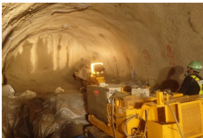
Figure 7: Spraying of back fill material.
