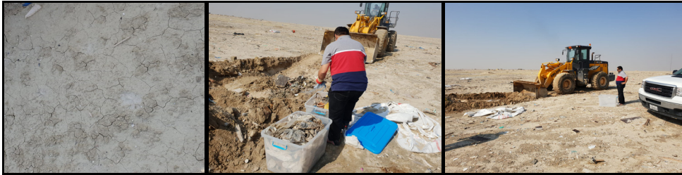
Figure 1: Pictorial depiction of the landfill mining process showing (left) soil top view of JAH landfill site, (middle) ditch excavation process at MAB, and (right) spade tractor operation/excavation of waste at MAB.
